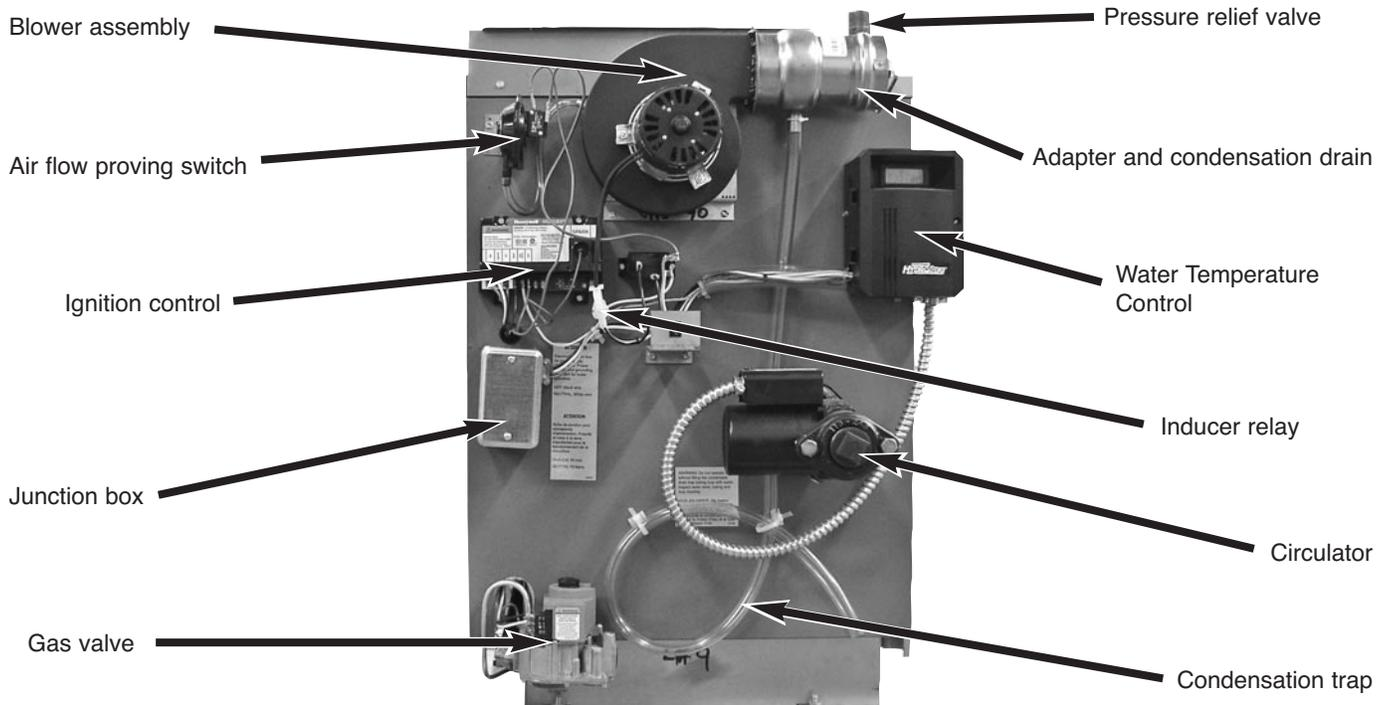
**Figure 1. Location and identification of parts**
